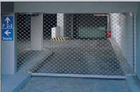
Security and ventilation in underground garages.
