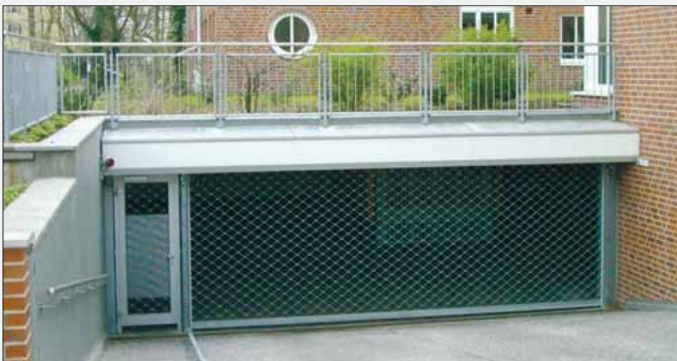
Roller grilles with side door in underground garages.
