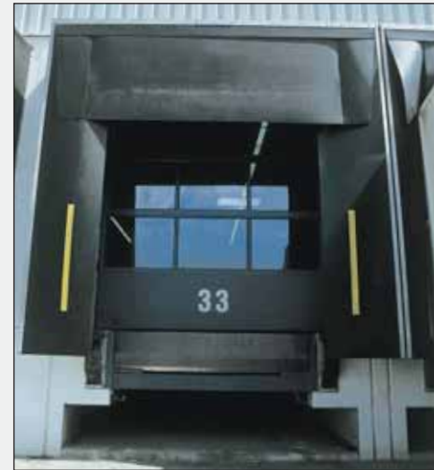
SLW sectional door for loading ramp.
