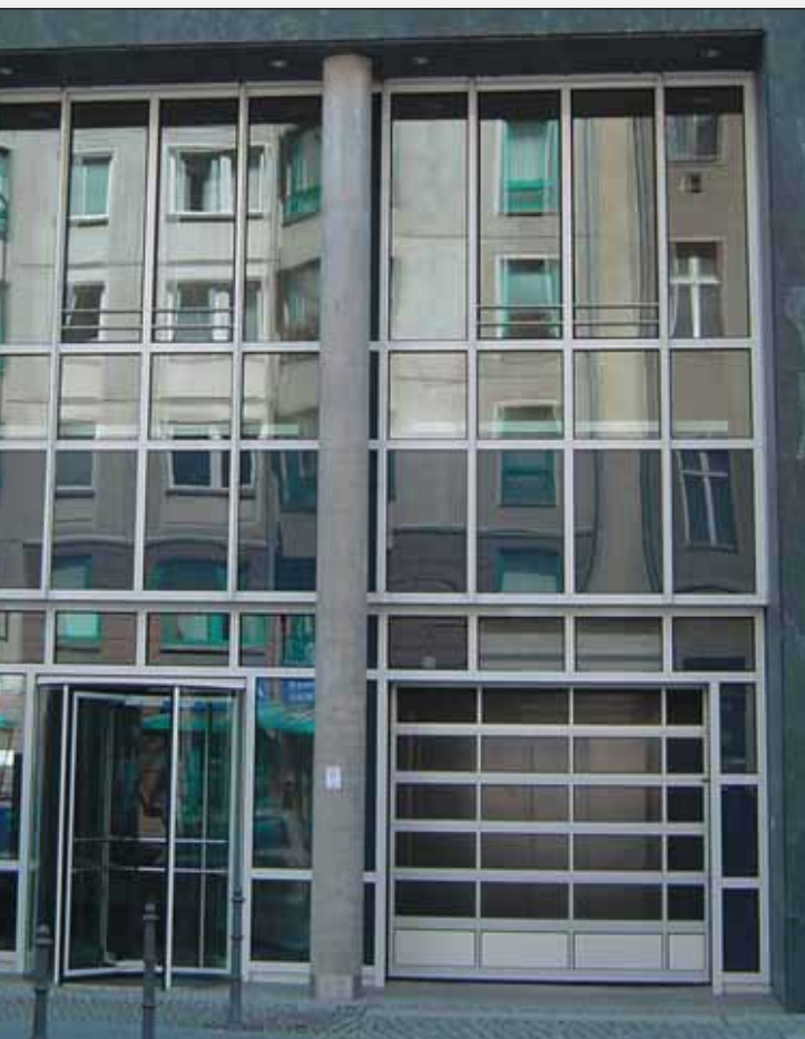
SL sectional door, optical integration into glass façade.
