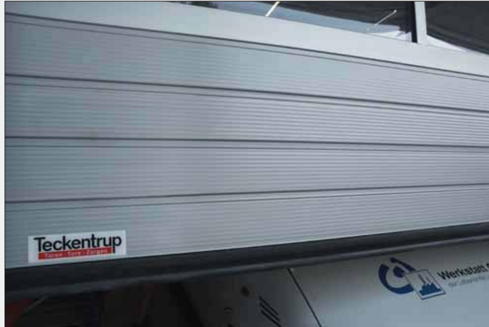
SLW sectional door, micro-profiled with glazing strip.
