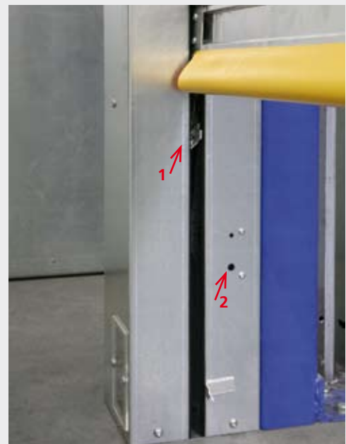
Pre-running safety photocell(1) and door line photocell (2) for high protection.
